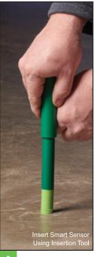
**<u>TIP:</u>** Check the L6 Smart Sensor prior to installation to ensure there is a properly functioning sensor that is giving a reading.
