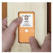
the floor plank into the rest of the floor system, make sure that no adhesives or other construction-related materials interfere with the underside of the Floor Sentry. Keep in mind that each side (both top and bottom) of the Floor Sentry contains a sensor. Be sure to note and record the location of the Floor Sentry installation for future reference.
